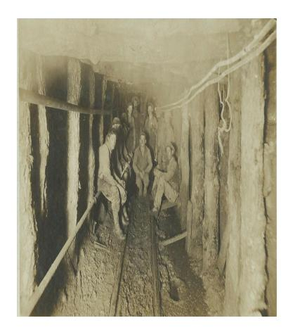
Above photo, from our archives, is labeled only, "Mifflin mines" on the back. This would have been a typical drift that miners, such as Ernest Miller would have labored in. Ore car tracks in the center and timber supports are visible as well as pipes to keep water pumped out.
